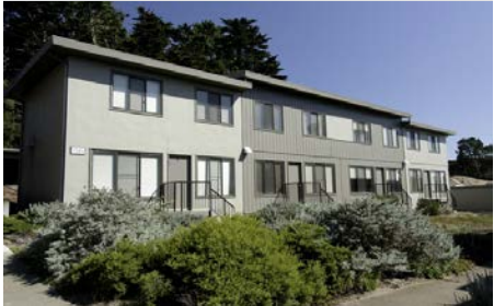
Baker Beach Rehabilitation Project San Francisco, CA
