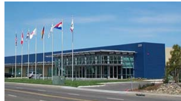
California Fuel Cell, West Sacramento, CA 1-story concrete tilt-up R&D Industrial Facility
