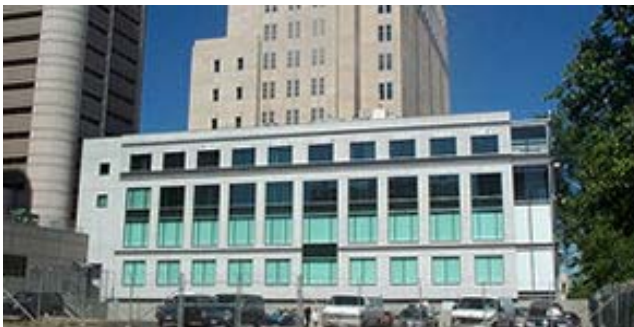
Hall of Justice, Sacramento, CA 4-story steel moment frame Class A Offices
