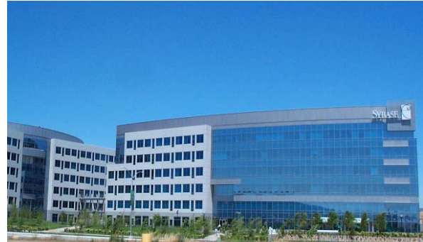
Sybase Corp Headquarters, Dublin, CA 6-story steel moment frame Class A Offices
