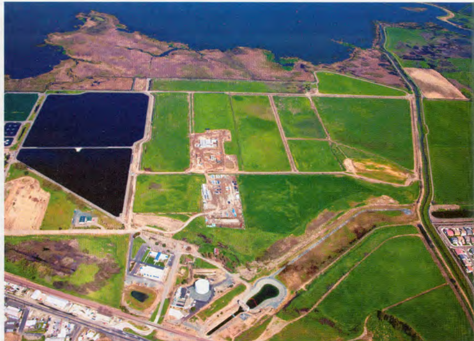
The Ironhouse Sanitary District's wastewater treatment plant project site is located in Oakley, Calif., less than 1,000 feet from the south shoreline of the Big Break Slough in the low-lying San Joaquin/Sacramento River Delta.
