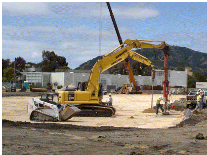
Fig. 2. Typical RAP installation equipment.
