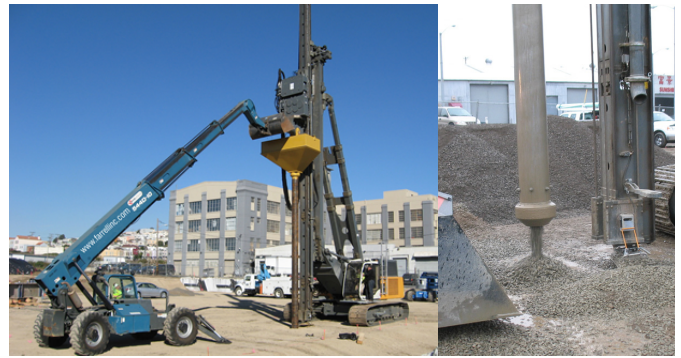
Fig. 2: Impact pier equipment with standard rammer head
