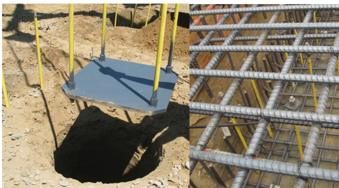
Fig. 1 RAP Uplift Bottom Assembly and Top Anchor
